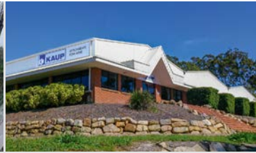
Production site Brisbane · Australia
